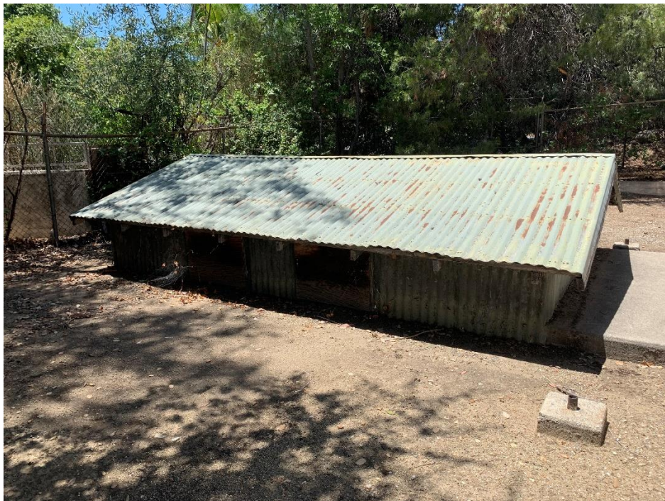
Figure 1. Existing Hydraulic Break Facility
