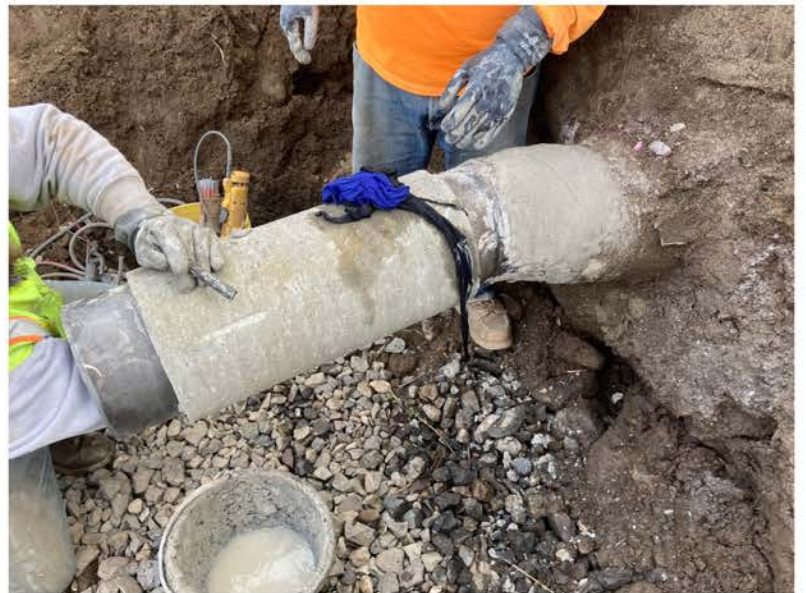
Frankish Tunnel Improvements - 2021
