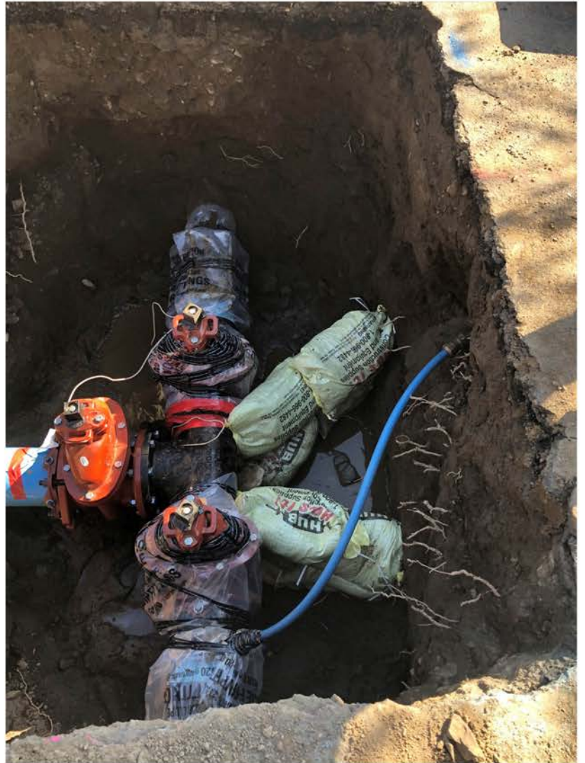
Euclid Crest Pipeline Replacement - 2021
