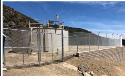
Holly Drive Tank Pad
