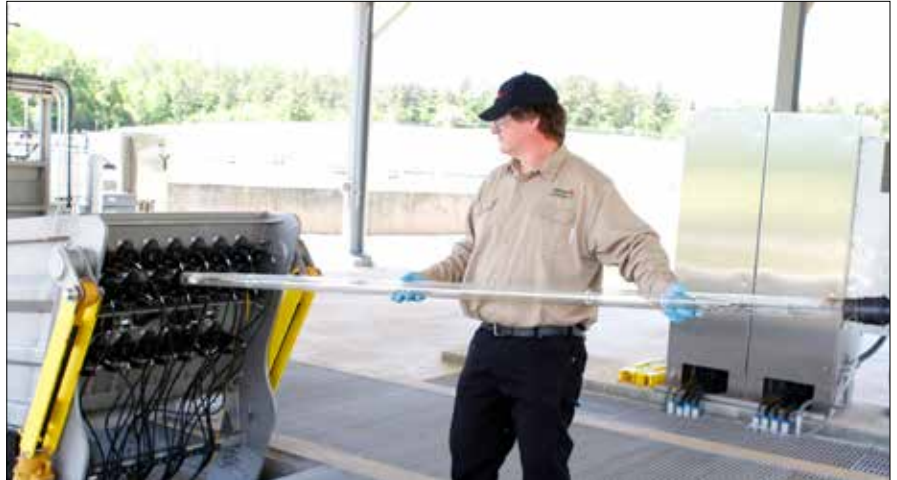
Routine maintenance is performed while banks are in the channel. However, when needed, banks can be raised by pressing a button and activating the ARM.
